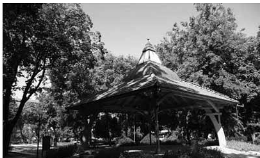
Wooden „Alltech” pavilion built at the former catholic church
