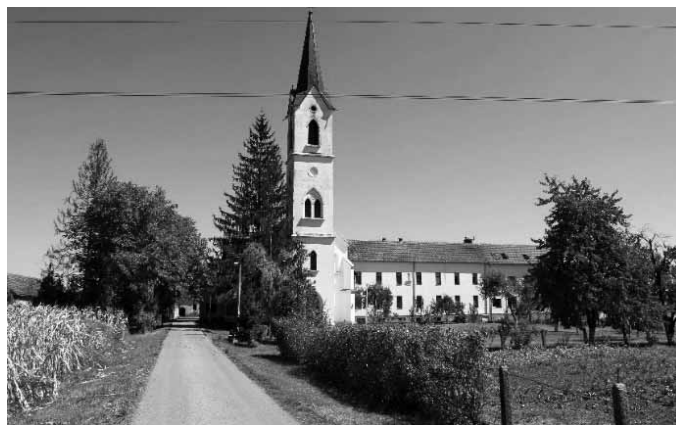
Convent with church in Marjanovac, Aleksandrovac; view from the west; present condition (Author's private collection. Photograph taken during August 2012)
